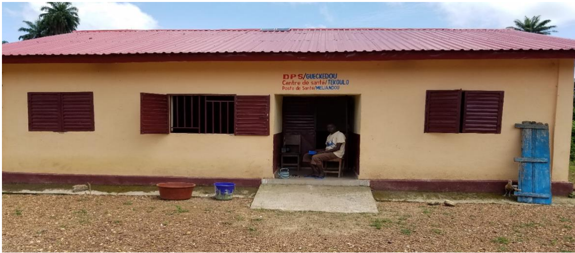
The renovated clinic in the village of Tana
